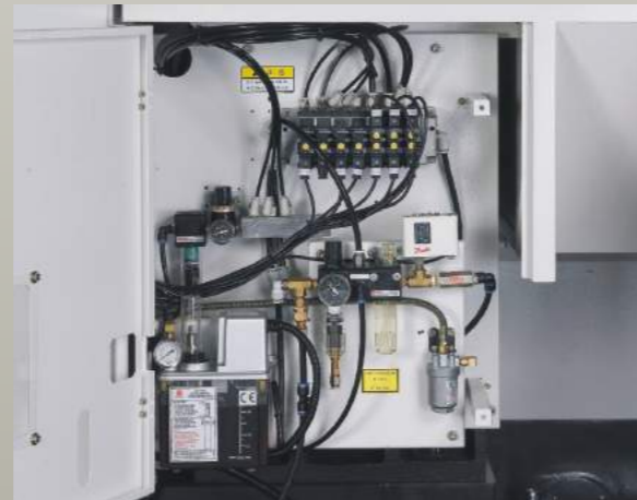
Hydraulic & Lubrication System(LU-620)
