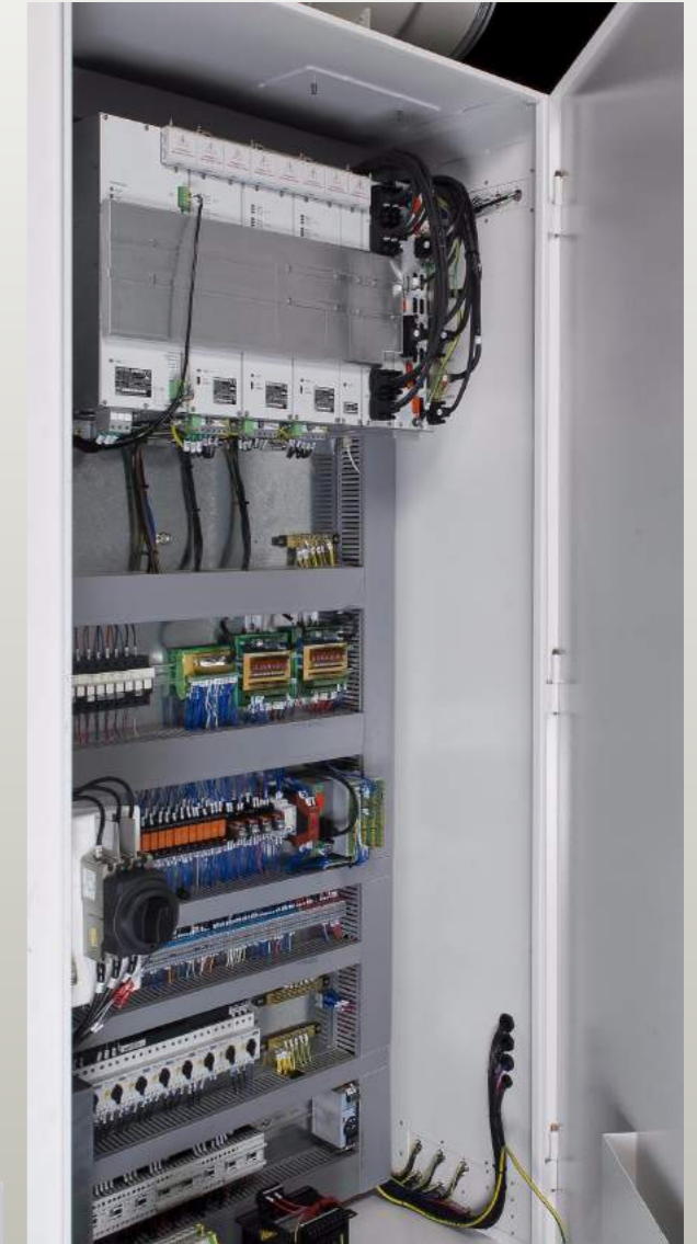
Electric System For Easy Maintenance
